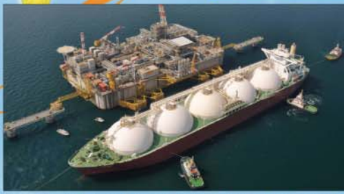
In August 2008, ExxonMobil Corp. delivered its first LNG cargo to the 8-4000-cu-meter (275-MBcu) Adriatic LNG regasification terminal 10 miles off Porto Levante, Italy. Making the delivery was the 135,000-cu-m LNG carrier Bahian. Adriatic LNG is the world's first offshore gravity-based LNG regasification terminal. The concrete structure stands in 85 ft of water, housing two LNG storage tanks, a regasification plant, and facilities for mooring and unloading LNG vessels. Adriatic LNG is jointly owned by Batar Terminal Ltd., a Batar Petroleum subsidiary, with a 40% stake, ExxonMobil Italiana Gas 40%, and Edison SPA 16%. (Photograph from ExxonMobil Corp.)
